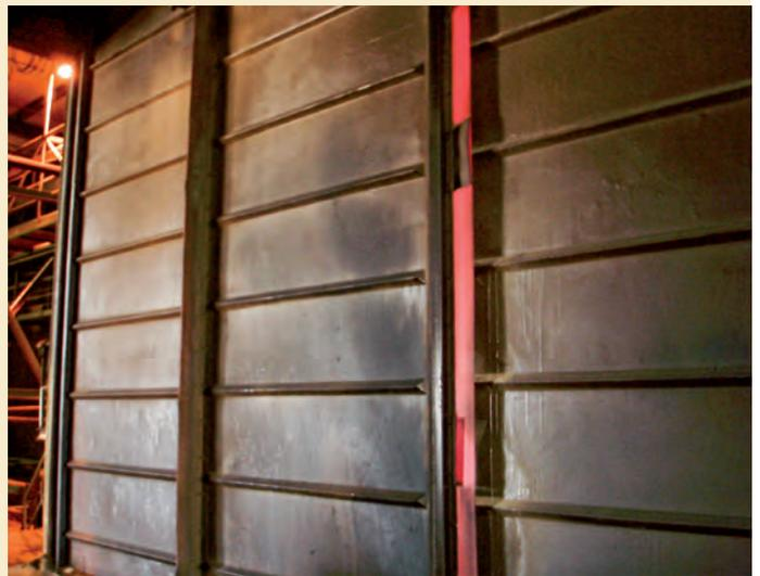
*After being surfaced with the waterproofing compound, the steel surfaces of the drying house have remained in good condition for three and half years. Normally, the surface material starts peeling off in large areas within a year.*
