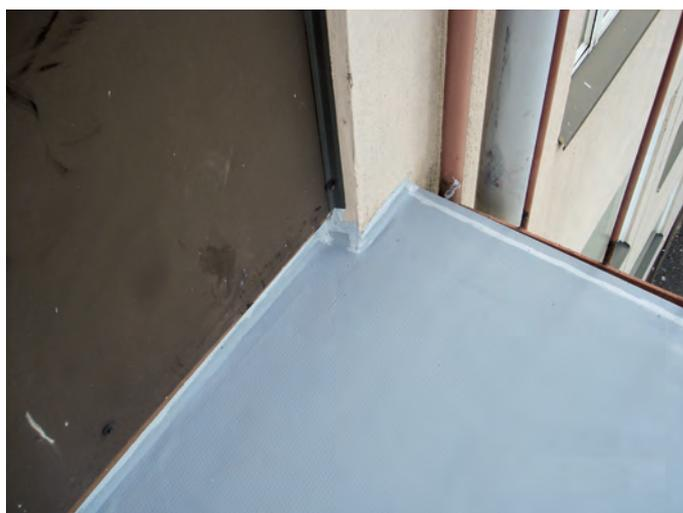
A balcony has been repaired by attaching a polypropylene-coated sheet on the balcony slab using Elastop.
