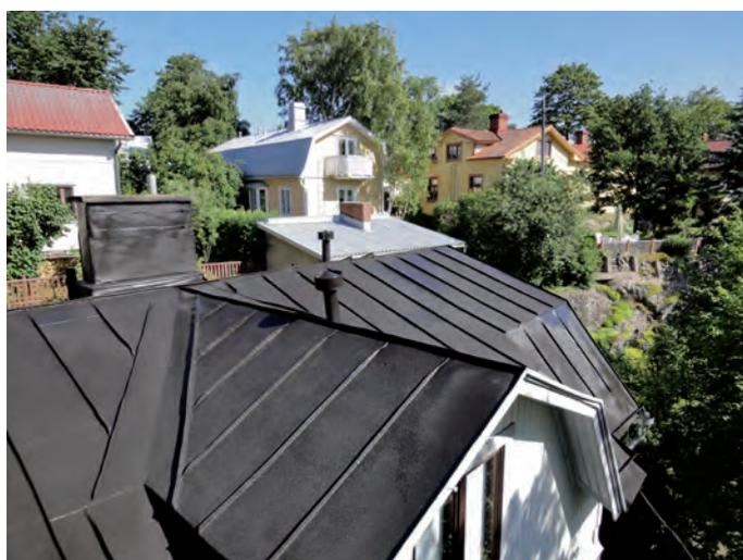
An old sheet metal roof has been repaired by spreading a thin layer (slightly more than one millimeter) of Elastop on it. The surface can be finished with paint.
