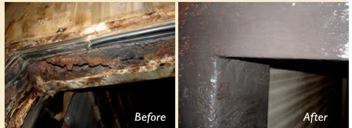
*A door frame made of structural steel has been repaired using Elastop waterproofing compound and a reinforcement fabric.*
